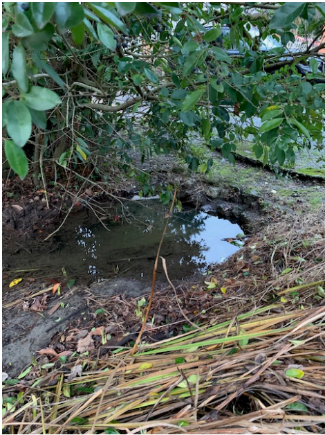
Culvert Discharge to open Ditch Point F
